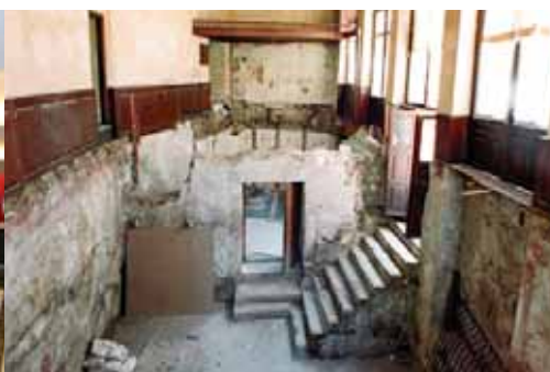
Underpinning of a listed building housing a Starbucks Coffee Plaka
