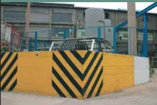
HALYVOURGIKI (EAF reactor foundation) Elefsina
