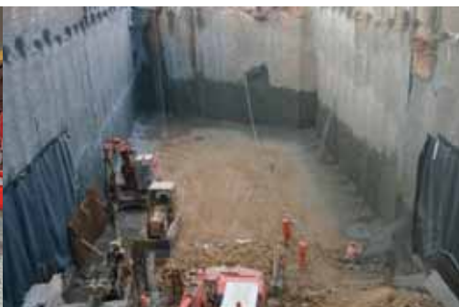
Foundations for EMVRYIKI DIMIOURGIA building Halandri
