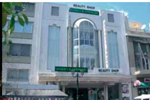
MARKS & SPENCER Former Capitol Cinema, Piraeus
