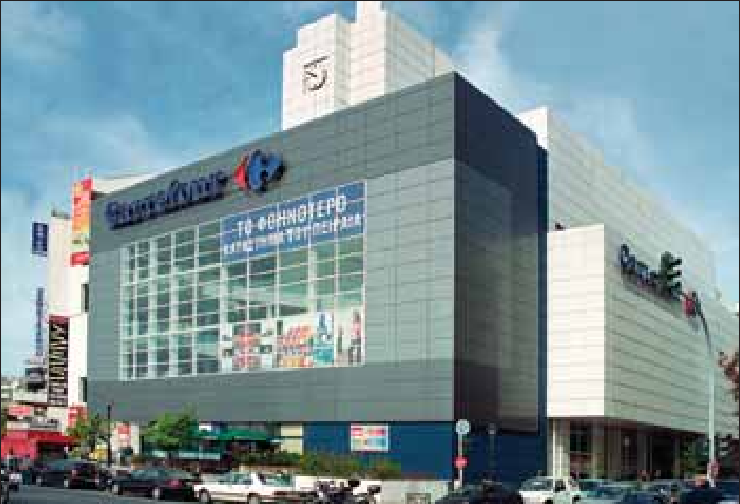
Expansion and renovation of CARREFOUR hypermarket Pashalimani, Piraeus
