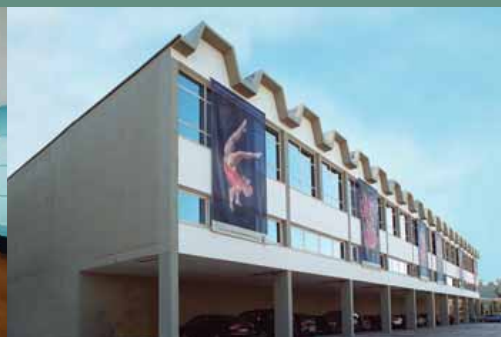
Maintenance work on façade of PIERCE COLLEGE Agia Paraskevi
