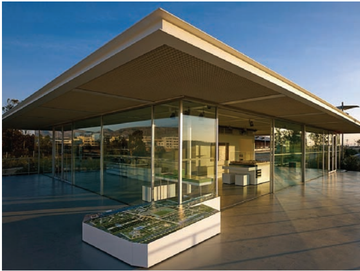
SNFCC Visitors' Centre - Neo Faliro, Attica
