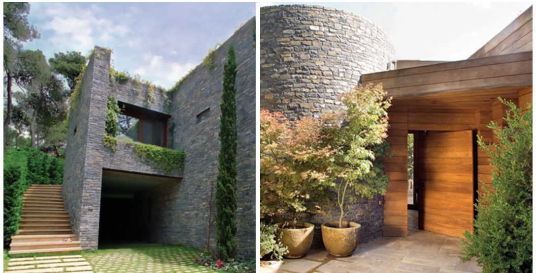
Residence - Ekali, Attica
